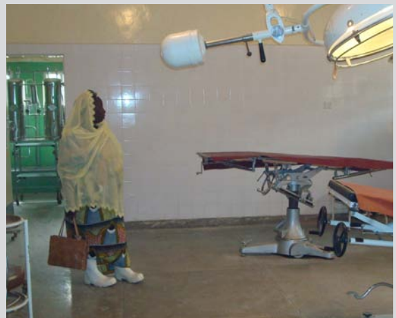
Old theatre finishes removed and replaced with more hygienic materials
