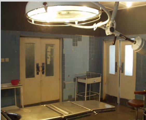
Old theatre finishes removed and replaced with more hygienic materials
